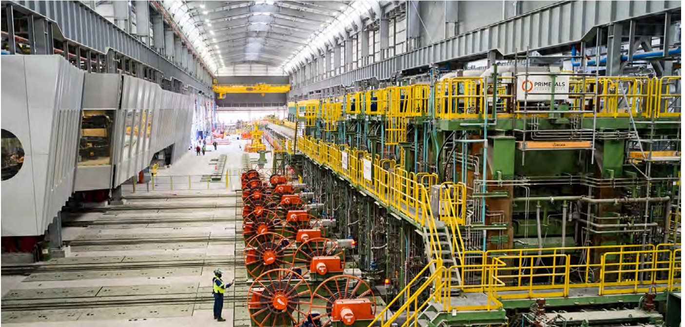
Pesquería New Hot Rolling Mill - The process of coil formation is carried out through hot rolling equipment.
